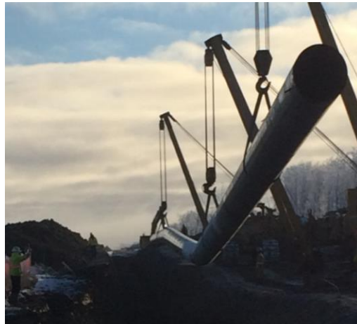
740 + 100 lowering pipe into ditch
