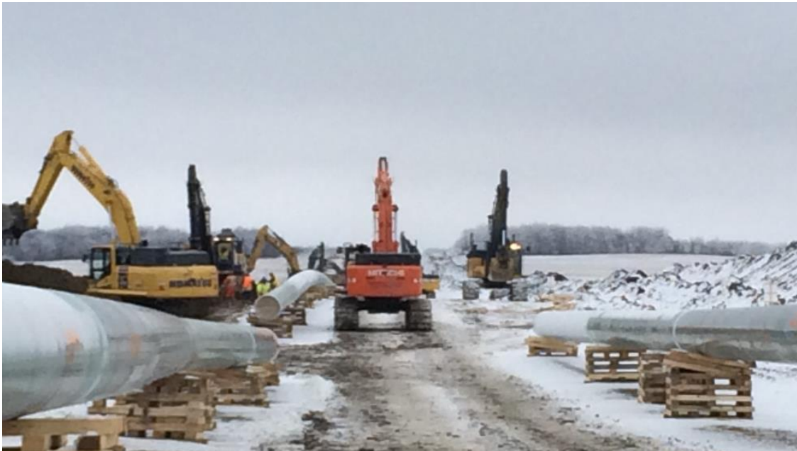
785 + 051 Track hoes excavating ditch line
