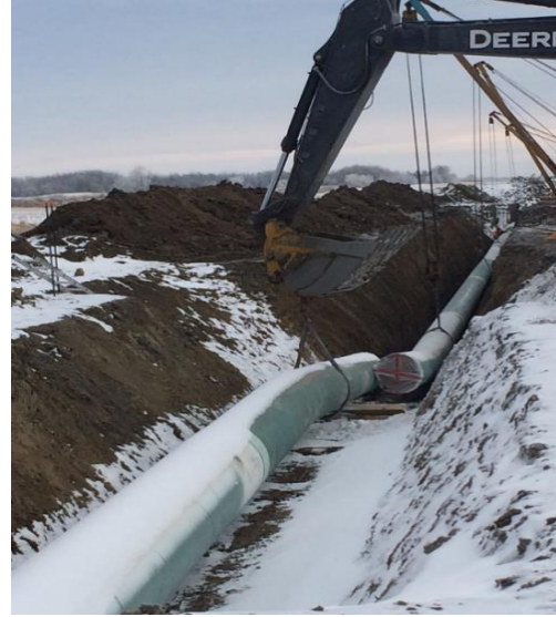
740 + 100 lowering pipe into ditch
