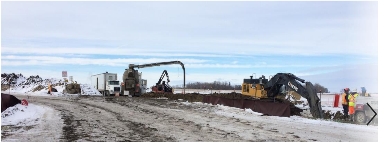
785 + 051 HD bore at access road
