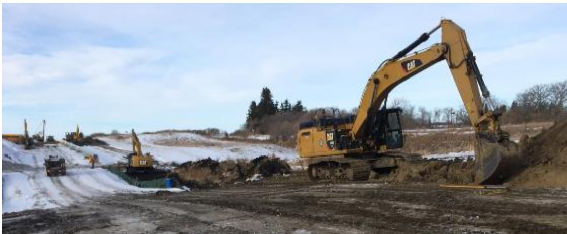
725 + 225 Wetland SK 771 Trachoes stripping top layer
