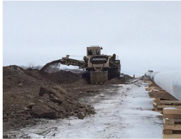
786 + 500 ditch wheel excavating ditch
