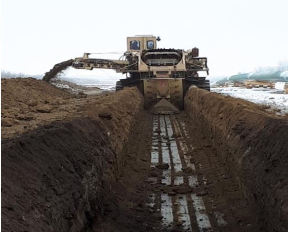
786 + 500 ditch wheel excavating ditch
