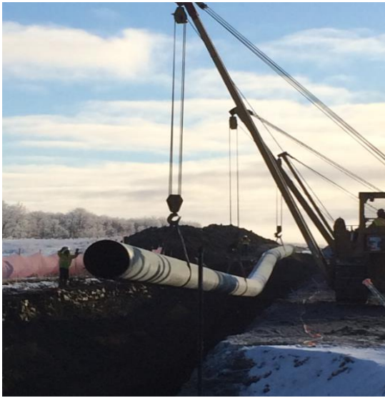
740 + 100 lowering pipe into ditch
