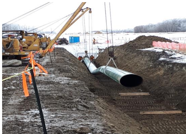
740 + 100 lowering pipe in ditch
